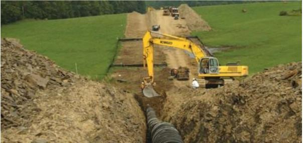
FIGURE 7: LAYING PIPE.
